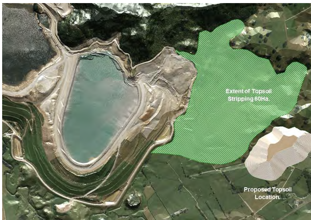
Figure 18-4: Preparatory Works for TSF3
