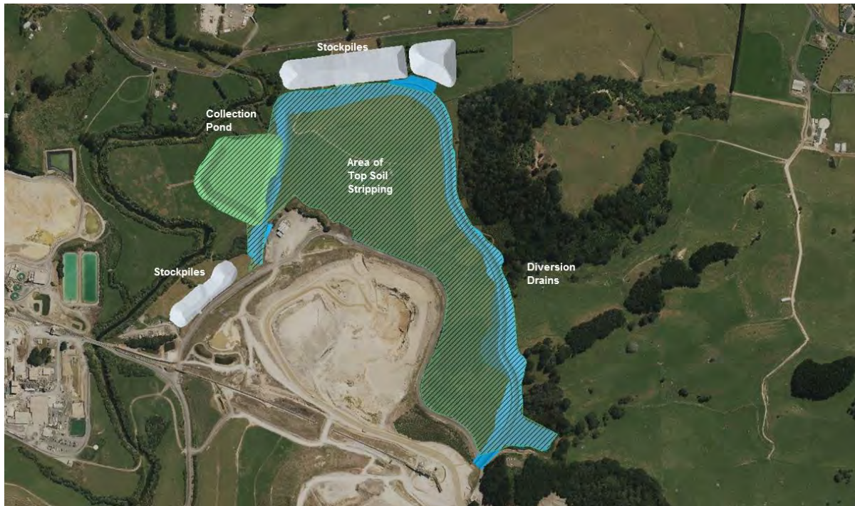
Figure 18-8: NRS Preparatory Works
