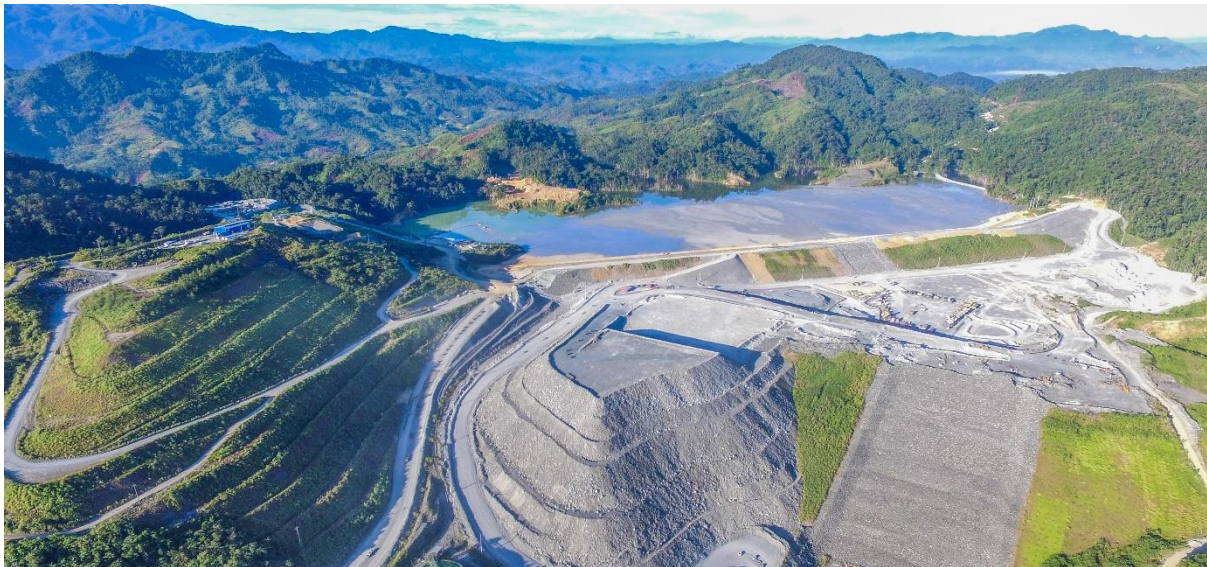
Tailings storage facility and waste rock stacks being progressively rehabilitated at the Didipio Mine
