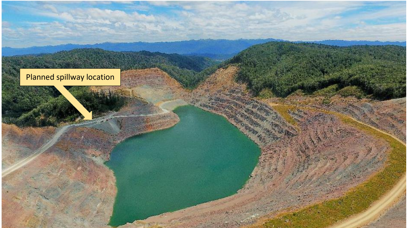
Figure 3 – Globe Pit Rehabilitation
