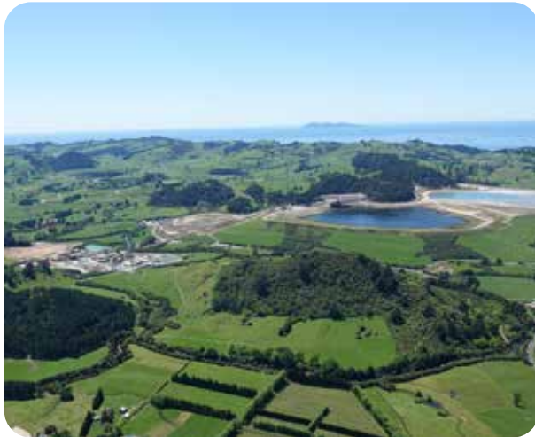
↑ Aerial view of Wahi Operation's tailings storage facilities, New Zealand
