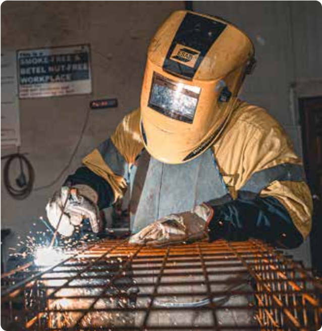
Process plant welder
