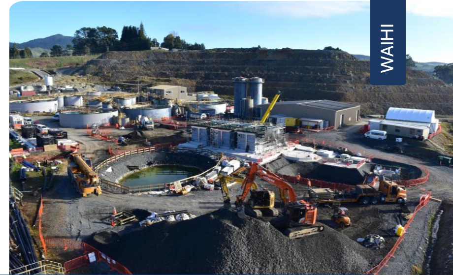
Water treatment plant – May 2026
