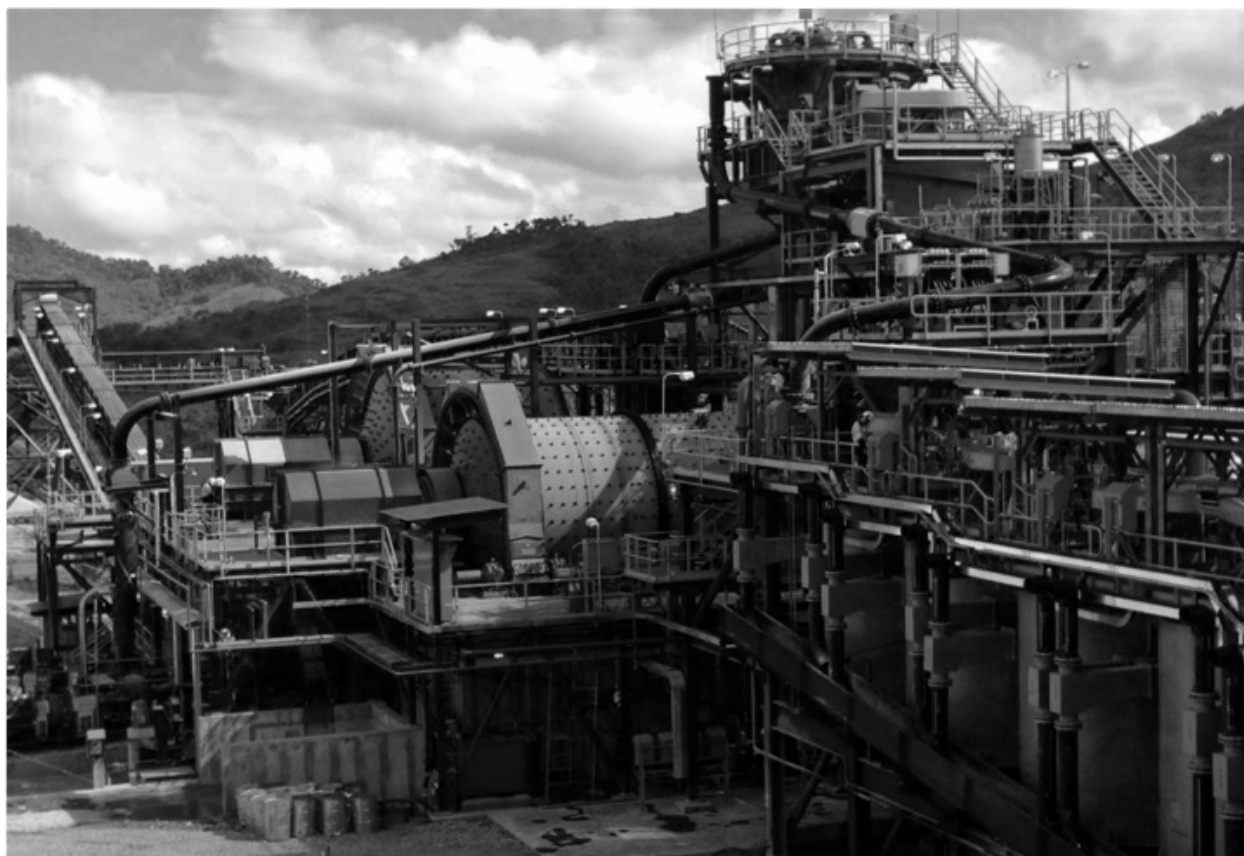
Figure 2: Completed Process Plant, December 2012
