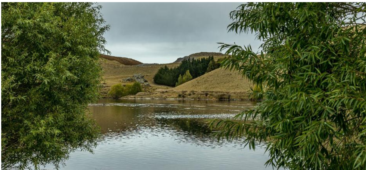
Lone Pine Dam at the Macraes Operation in New Zealand.
