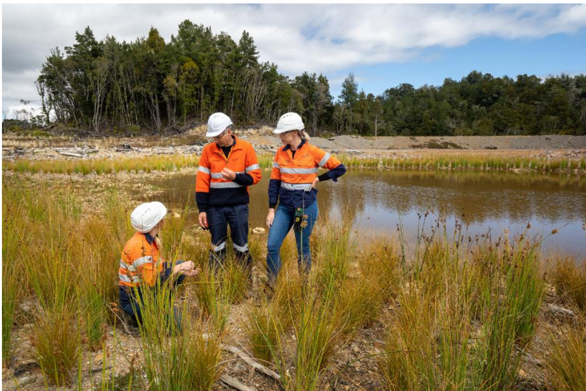
An engineered wetland at the former tailings storage facility at the Reefton Restoration Project in New Zealand. The wetland is designed to ensure long-term sediment control of the lake's discharge.
