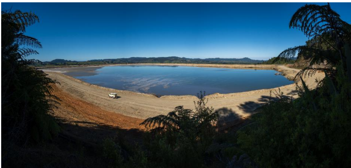
Tailings storage facility at our Waihi Operation in New Zealand.
